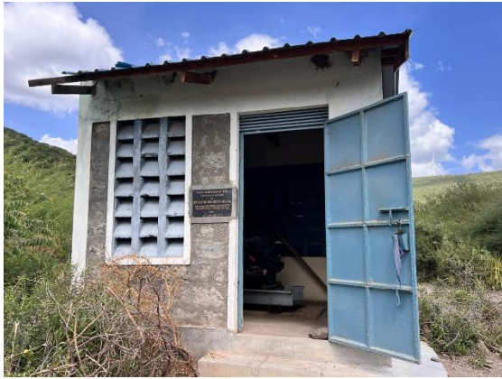
View of the Generator House
