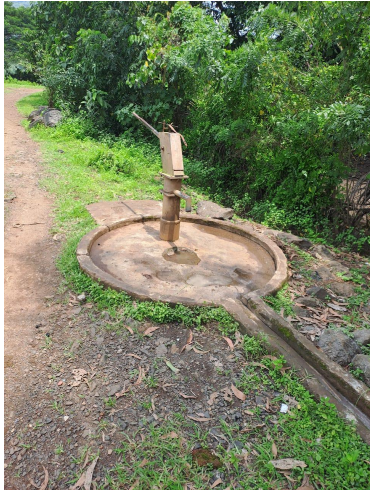
Existing Bore well
