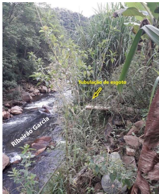
Effluent discharge directly into the Garcia stream
