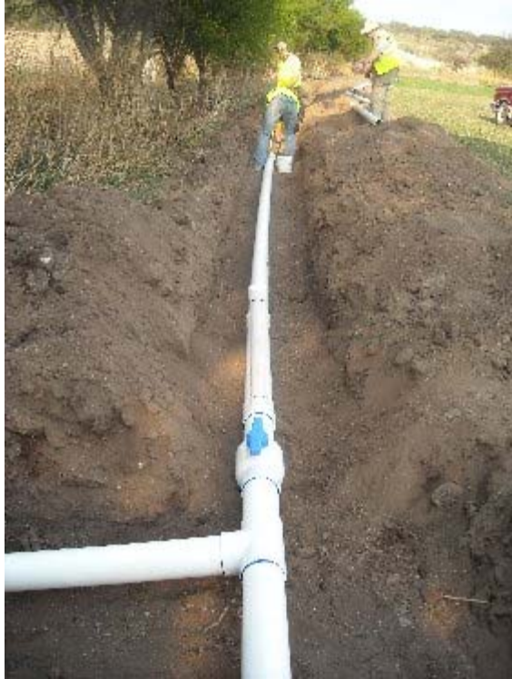
Figure 2 - Pipeline Installation
