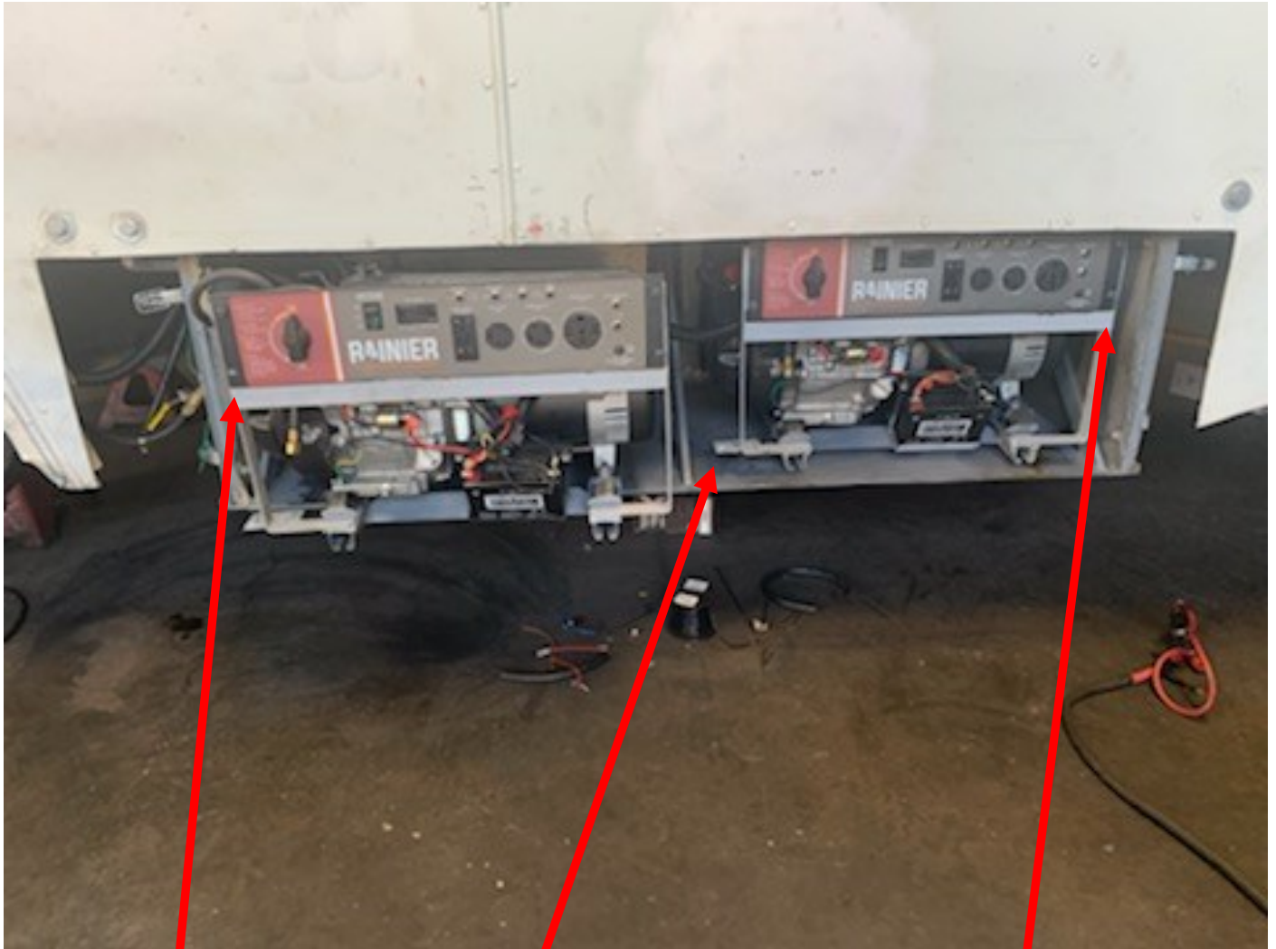
Generator cavity & cages
