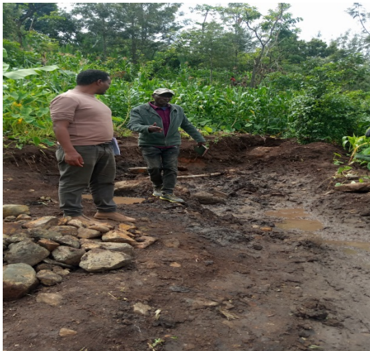
Site Clearance at Tulicha
