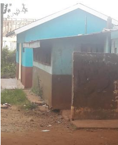
In the foreground the old latrines in the background the new CDF 4 cubicle construction for lower primary
