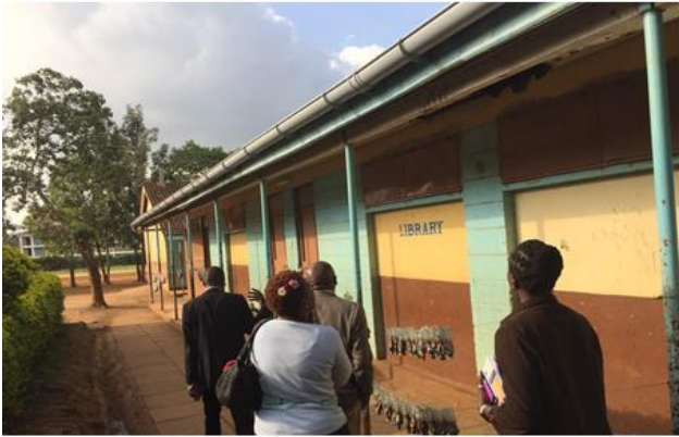
Rainwater roof harvesting- the computer lab
