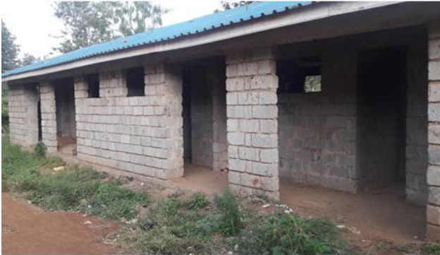
Stalled 24 cubicle flash type toilet construction project by LASDAP
