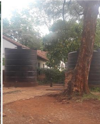
Water Storage Tanks
