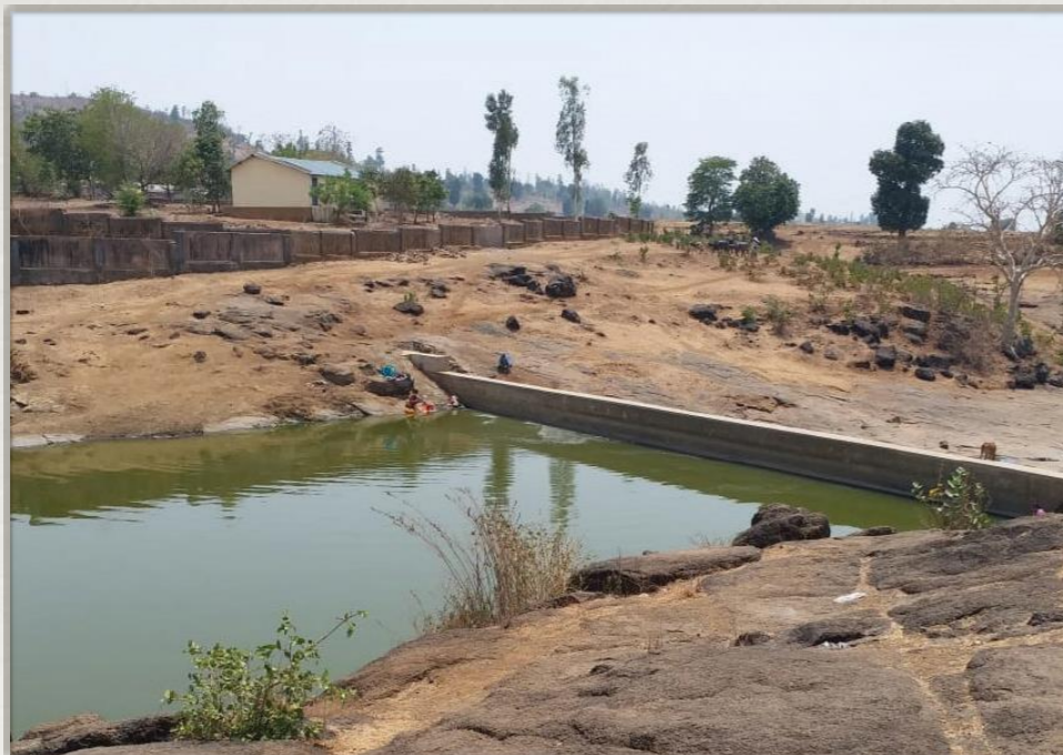
Check dam in Thane district - benefiting 25,000 people
