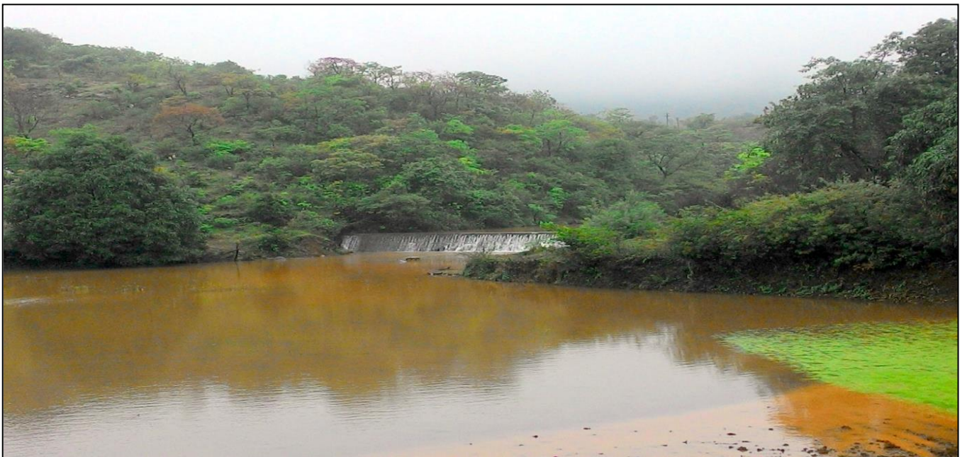
Figure 3: Damaged check dam
