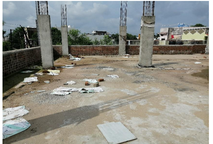
Proposed Training Centre under construction
