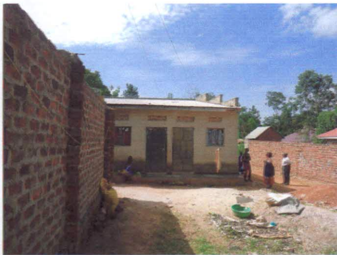
The buildings to be converted into a Health Unit
