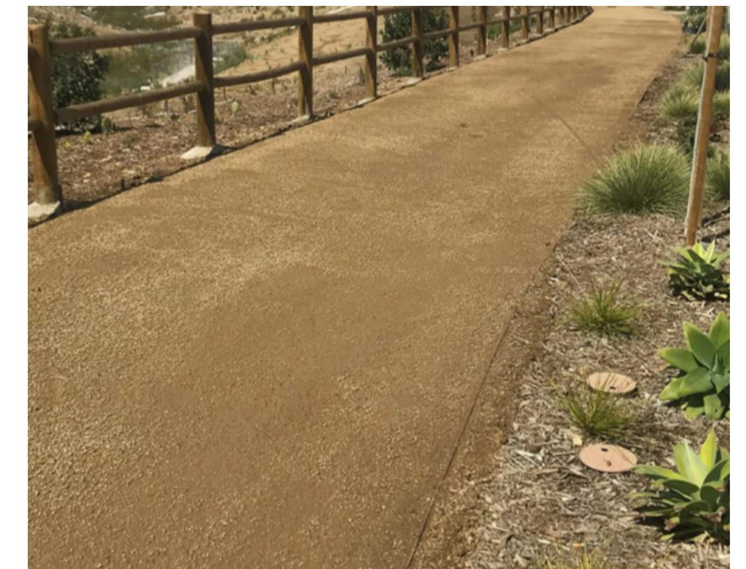
Stabilized Decomposed Granite Paving (D.G.) with Permaloc Aluminum Edging
