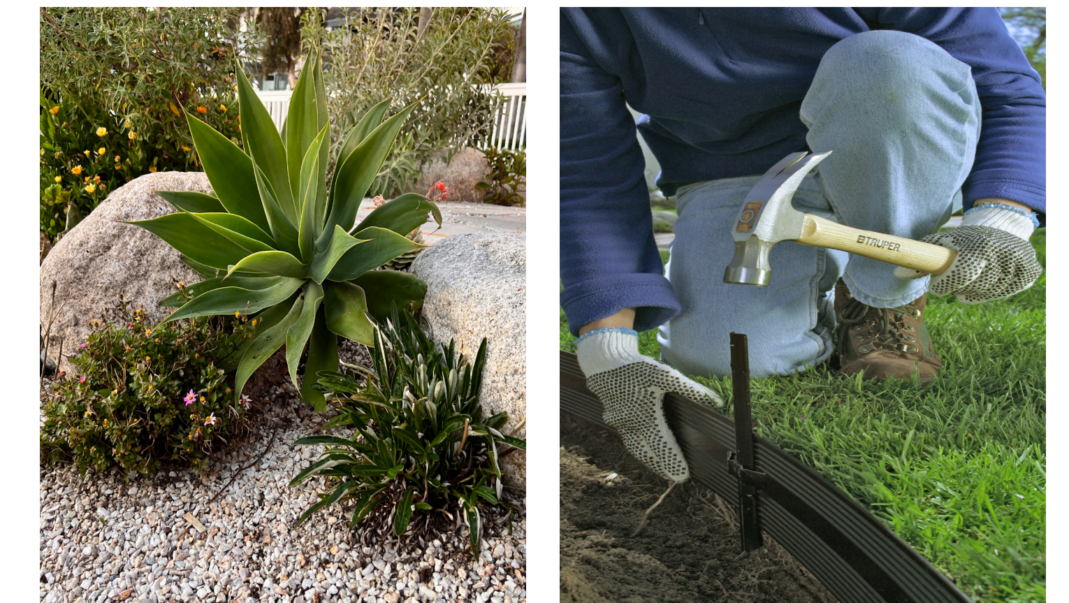
Stabilized Decomposed Granite Paving (D.G.) with Permaloc Aluminum Edging
