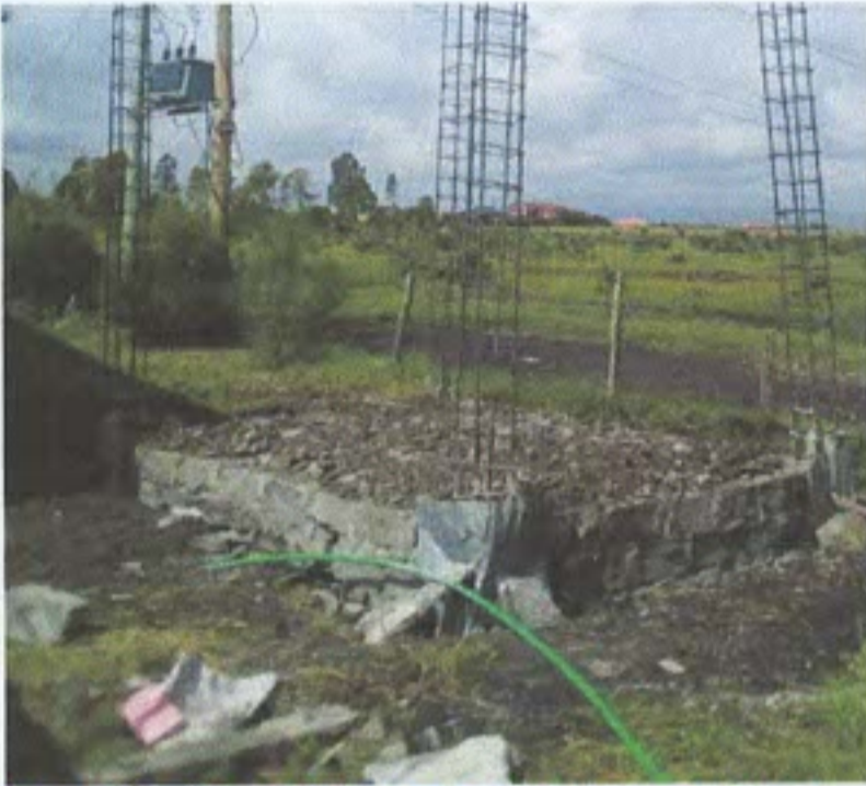
Figure 2 - Gantry foundation walls and slab
