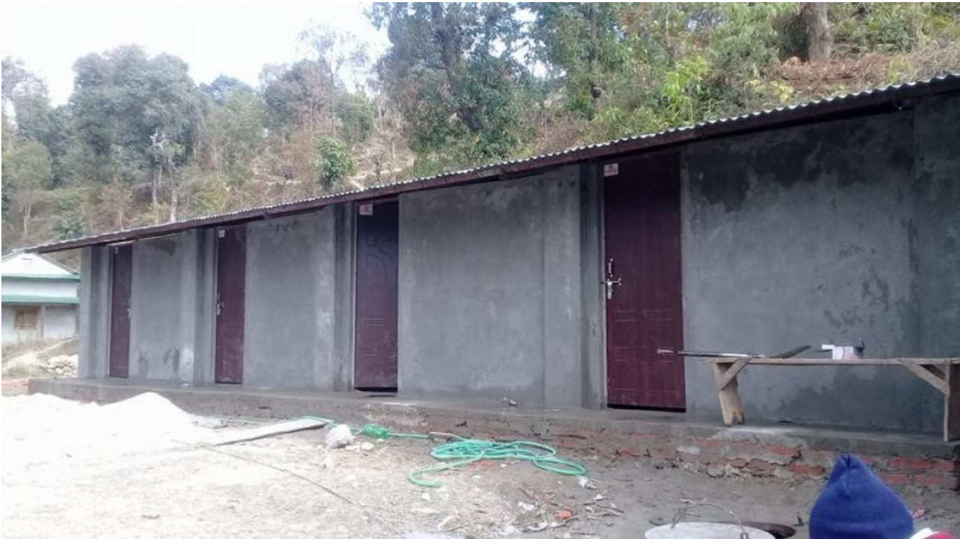
Refurbished school with stucco applied.
