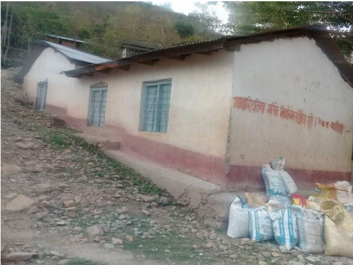
Construction materials on site.
