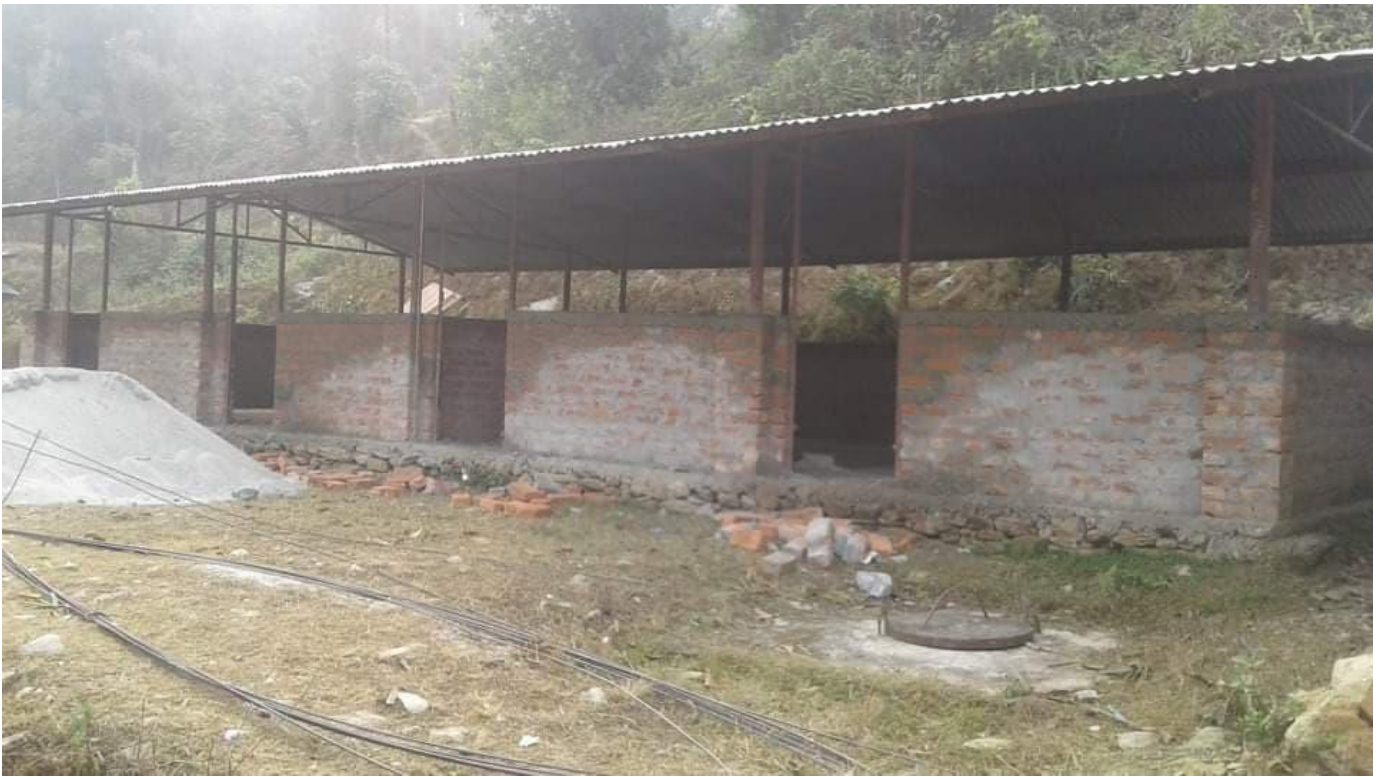
Lower wall brick.
