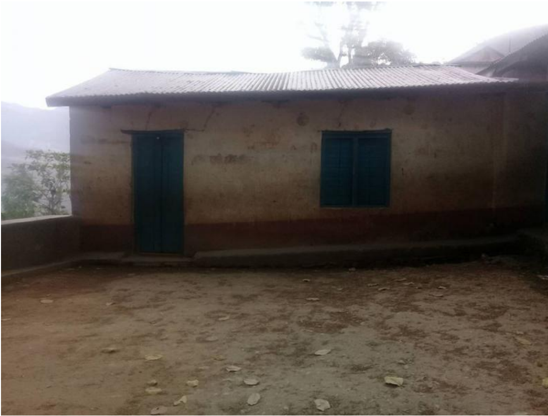
Ramechhap School before reconstruction.
