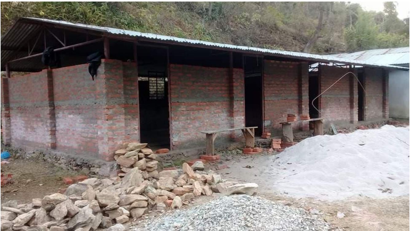
More views of brick structure nearly complete.
