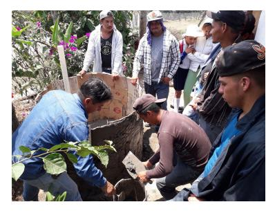
Our ferrocement tank training in the community of Plan del Hormiguero (above). The final rainwater tank (right) complete with a gutter system to collect rainwater directly from the roof.
