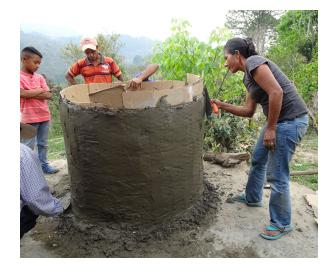
members have access to rainwater collected from their own roofs, but community members take part in the construction of the cisterns, learning new skills in ferrocement (a type of thin cement, that is supported by a thin layer of wire, and can be applied to any shape or size).
