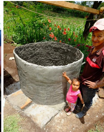
128 of 1,200 installed to date
