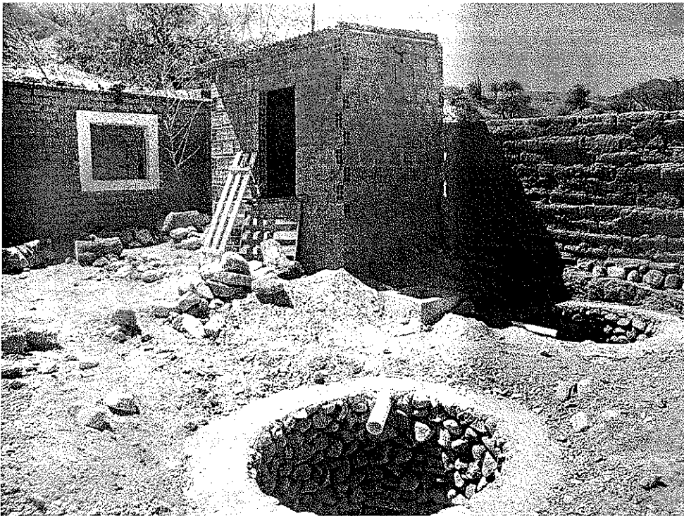
Two examples of completed bathrooms: both are constructed from adobe bricks.
